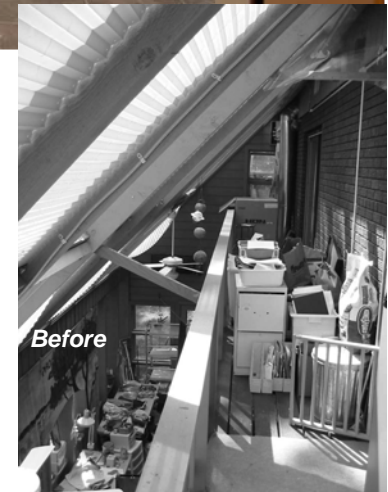
The old greenhouse with failed glazing and no views to the site.
