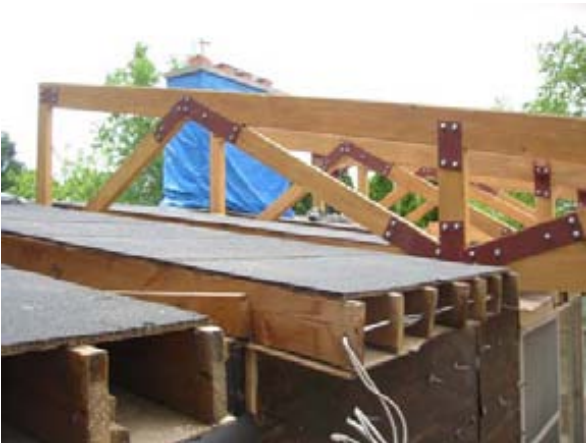
Sliding the new trusses into slots in the old roof.
