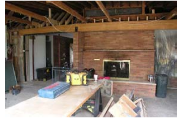
Demolition of the old ceiling, new exposed beam
