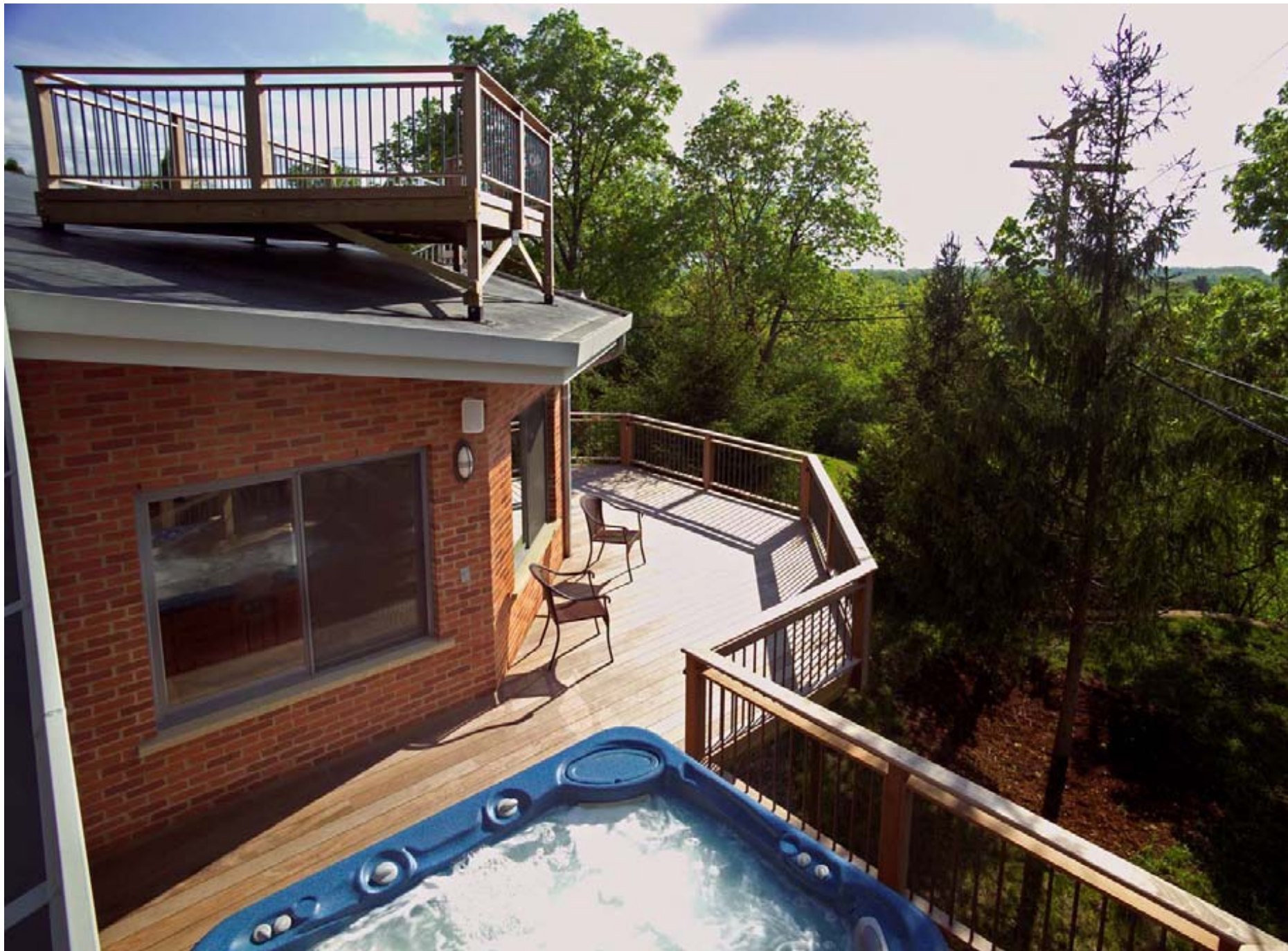
Two levels of decks are oriented to the incredible views of the horizon and the sky above. All decking is made of Ipe. Railings made of Ipe and round aluminum balusters.
