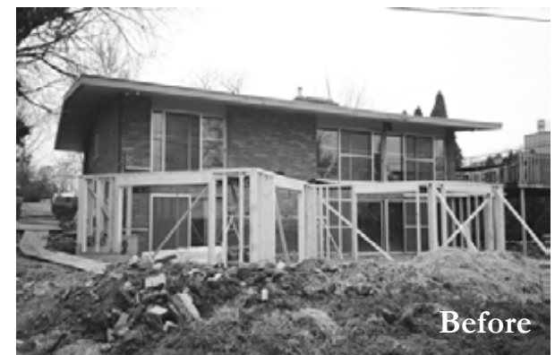
The old rear elevation can be seen as framing begins
