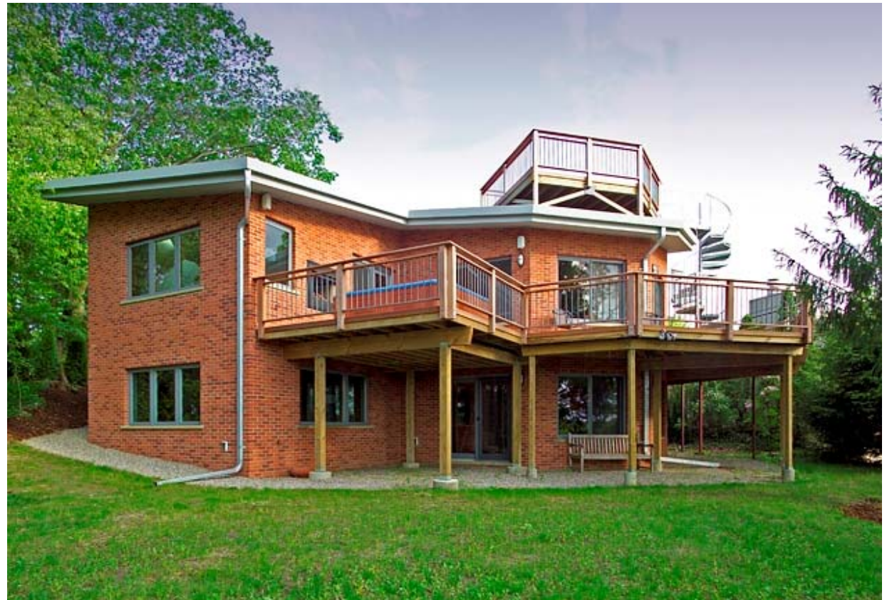
The rear elevation is all new with multiple levels a ‘winged’ roof plane. Note the rooftop star-gazing deck.
